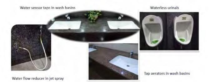
Photograph 7: Sensor based Taps at MIAL
